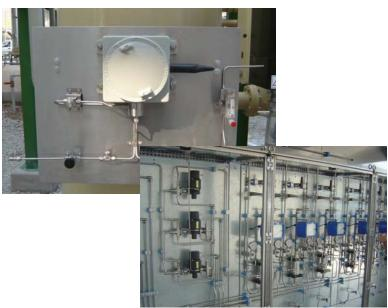
Our customized sampling products are designed and built for various specific requirements. Most of our systems are focused on the petro-chemical industry and power plant.
